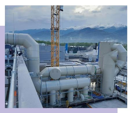
John Cockerill supplied gas scrubbers to treat discharges from a new French plant of a semiconductor manufacturer.
