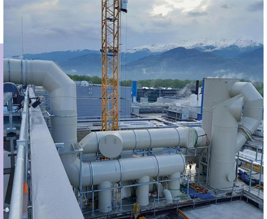
John Cockerill supplied gas scrubbers to treat discharges from a new French plant of a semiconductor manufacturer.
