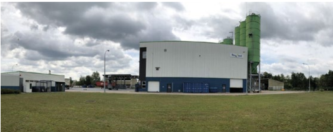
John Cockerill increased Resolest's wastewater treatment capacity.
