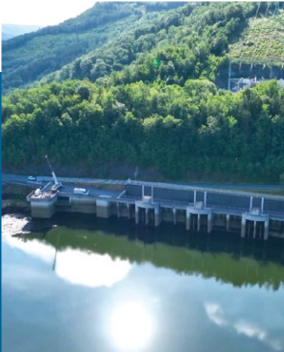
Renovation of the Revin hydroelectric dam (France).
