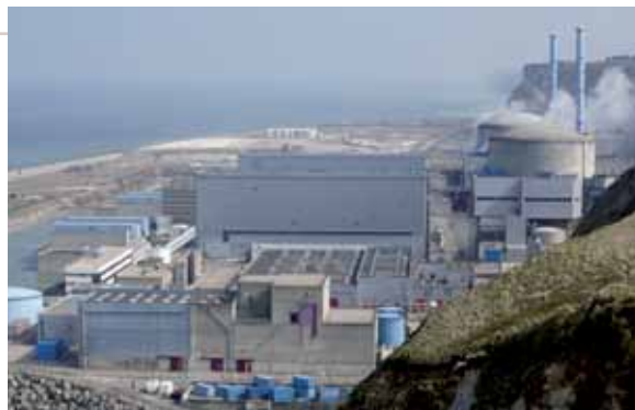
The proliferation of fouling organisms like, microbes, algae and mussels progressively reduces the heat transfer efficiency, and eventually leads to the clogging of the cooling water piping circuits of coastal industries and power plants.
