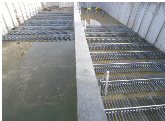
Particularly well-suited to increasing the capacity of existing wastewater treatment plants, the reconfiguration of the aeration basins is a key element of the BeFlow® AGS process, allowing to double treatment capacity
