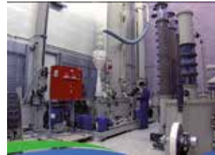
Pilot hall of more than 200 m 2
