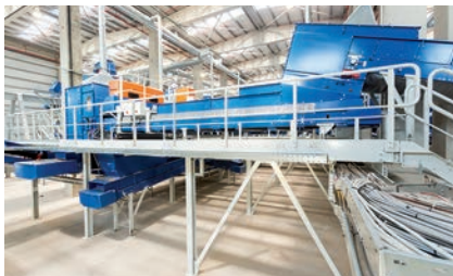
Sorting center Wastes recycling
