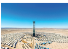
Solar Tower Receivers & Steam Generators
