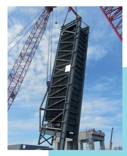
John Cockerill Energy modular designs (shop fabrication maximized as per Customer needs), such as the M100, help to minimize field labor construction works and meet challenging deadlines
