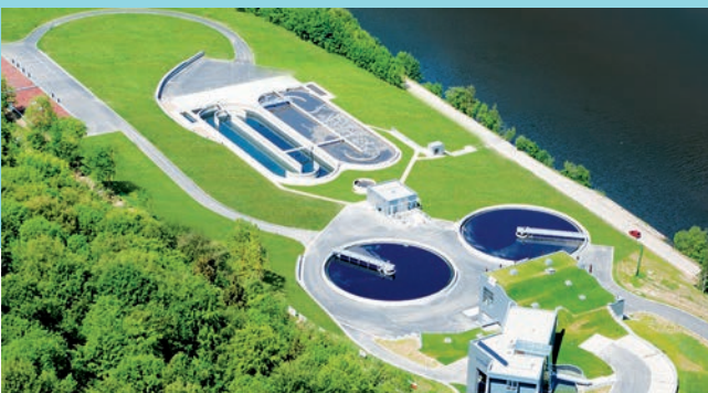
Municipal wastewater treatment plant, 93 100 PE (Namur, Belgium)
