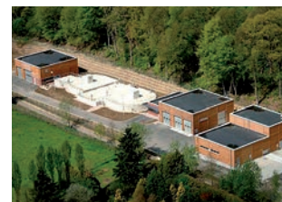
Wastewater treatment plant, 13 000 PE (Louvain-la-Neuve, Belgium)
