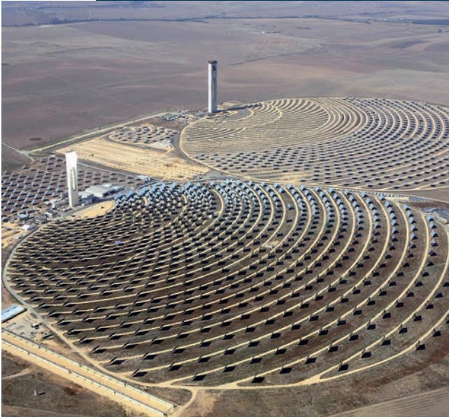
Solar thermal power plant
