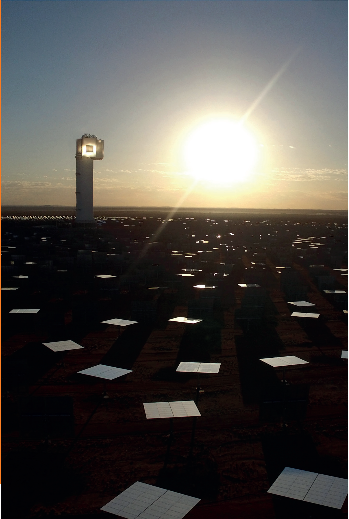
The central tower solar thermal plant of Upington (South Africa) equipped with a John Cockerill receiver
