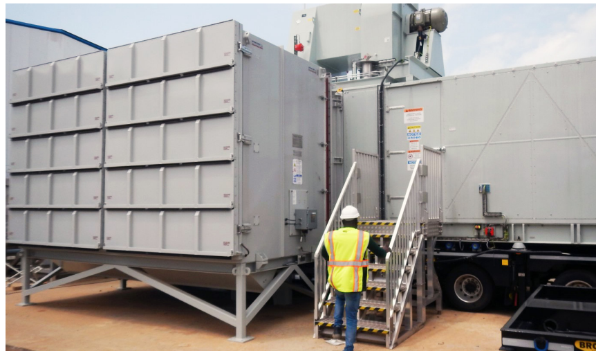
Truck Mounted Gas Turbine TM 2500+ at site.
