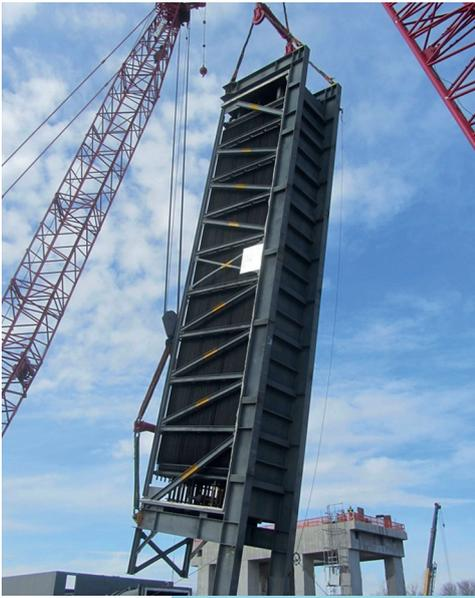
John Cockerill Energy modular designs (shop fabrication maximized as per Customer needs), such as the M100, help to minimize field labor construction works and meet challenging deadlines
