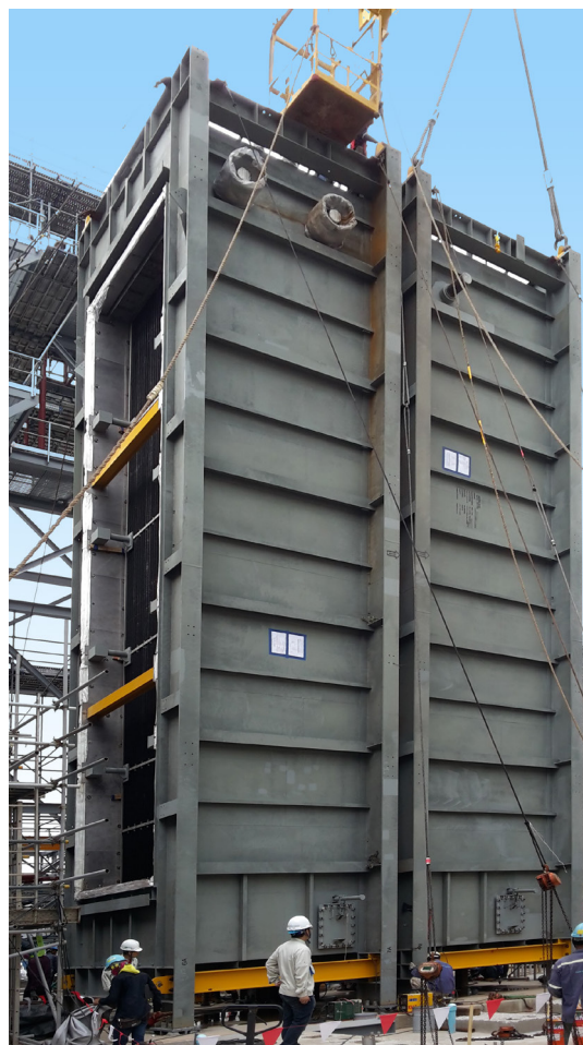
The Modular Box design enables a faster assembly of the boiler.
