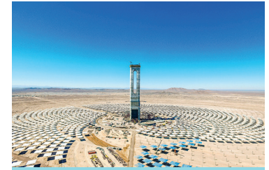
Solar Tower Receivers & Steam Generators
